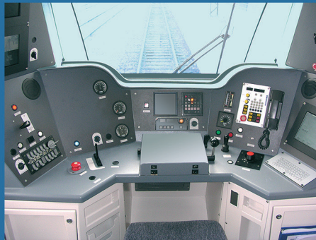
Railway control station.
